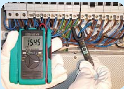
Measuring current in a Switchboard
